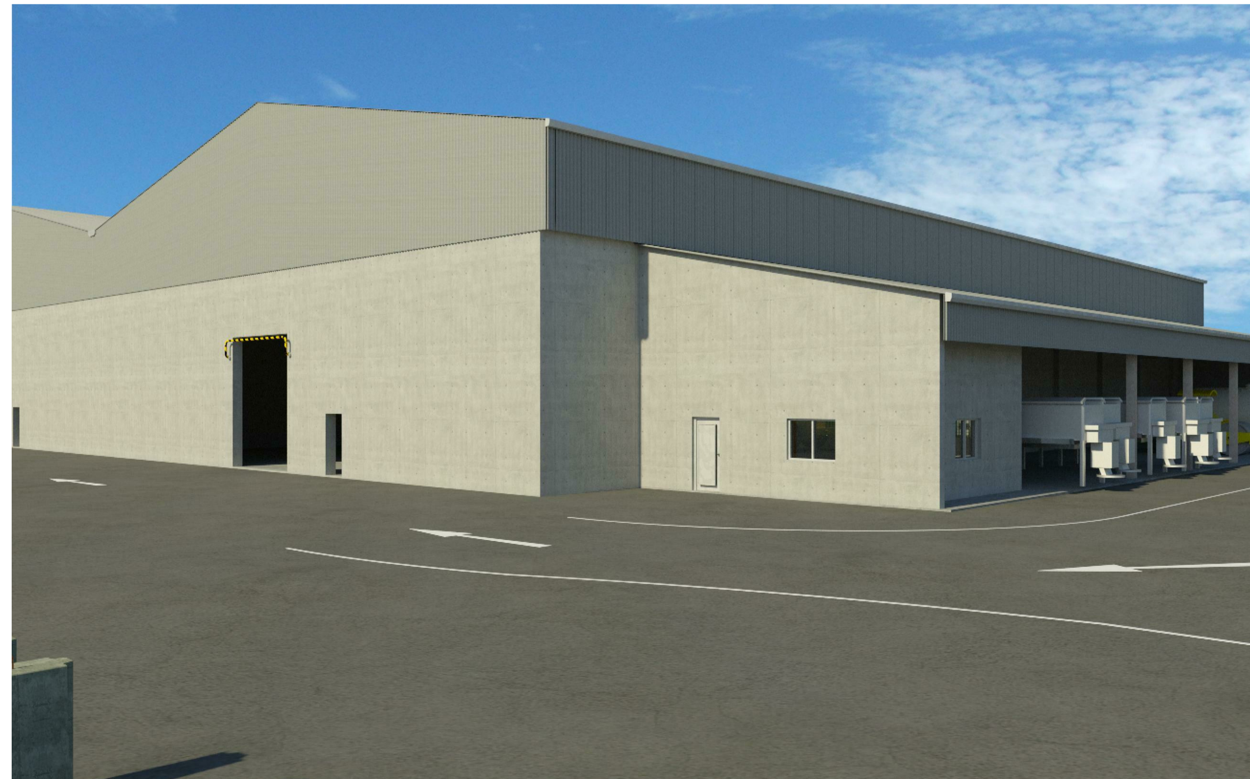
SALT BARN VIEWED FROM CHIP STORE AREA
